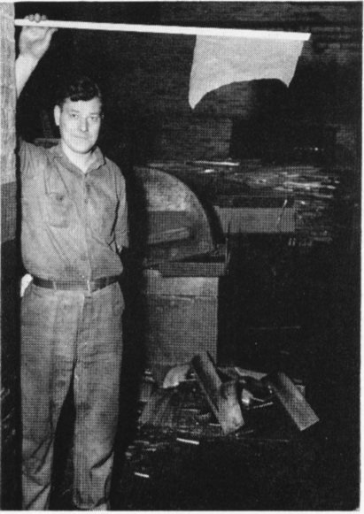
Charles Pranulis, of the North Mill, pulls down the red flag signaling "danger ahead" in the vicinity of a hidden work hazard in the Mill.
